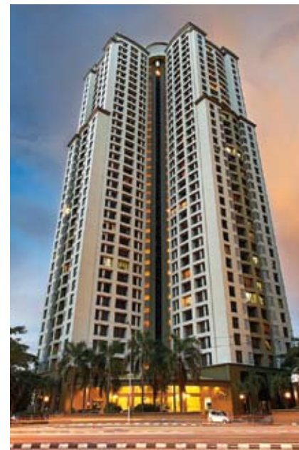
Vista Damai KLCC, Kuala Lumpur
